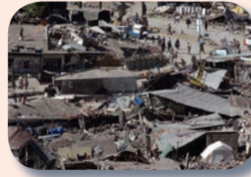
Unimaginable destruction caused by the massive earthquake in Pakistan.
